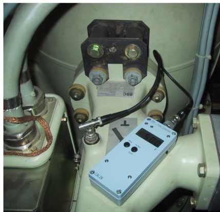
Calibration impulse generator connected to an earthing switch
