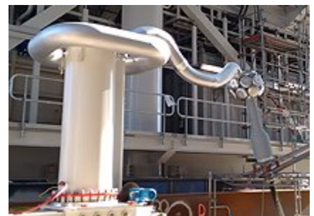
Fig. 13: Site acceptance test (SAT) on 220 kV cables according to IEC 60267
