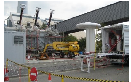
Fig. 17: Preparation for a 3-phase induced and voltage test
