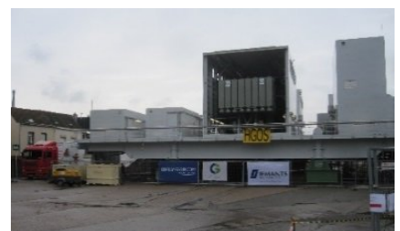
Fig. 14: 24h soak test on the HV cables of an offshore wind turbine substation
