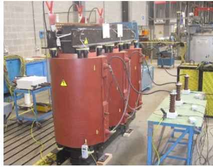
Fig. 21: 3-phase induced PD measurement on a dry type transformer
