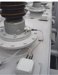
For manufacturing a custom made bushing adapter, Power Diagnostix needs the dimensions of the bushing's test tap. We have created a document to help our customers determine the most important dimensions.
