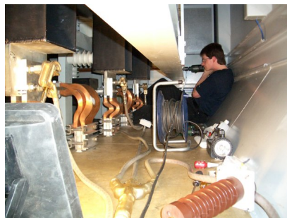
Installing couplers on site
